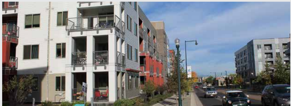
A VARIETY OF HOUSING IS APPROPRIATE ALONG BROOKS UP TO 50 UNITS PER ACRE
